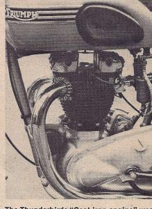
The Thunderbirds "Cast iron engine" was capable of terrific acceleration, with a power output of 34 HP at 6000 rpm and a strong torque curve. Bore and stroke measured 71 x 82 mm, and compression ratio was 7 to 1.
