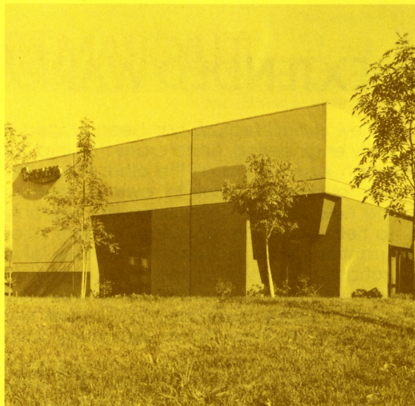
TMA's New Headquarters in Placentia, Calif.
